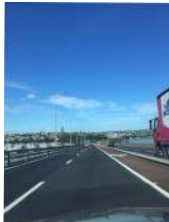
Empty roads on a trip across the bridge
