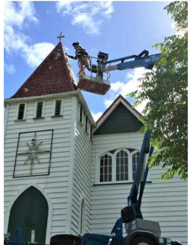
Peter Linnell repairing the steeple - St Paul's Church
